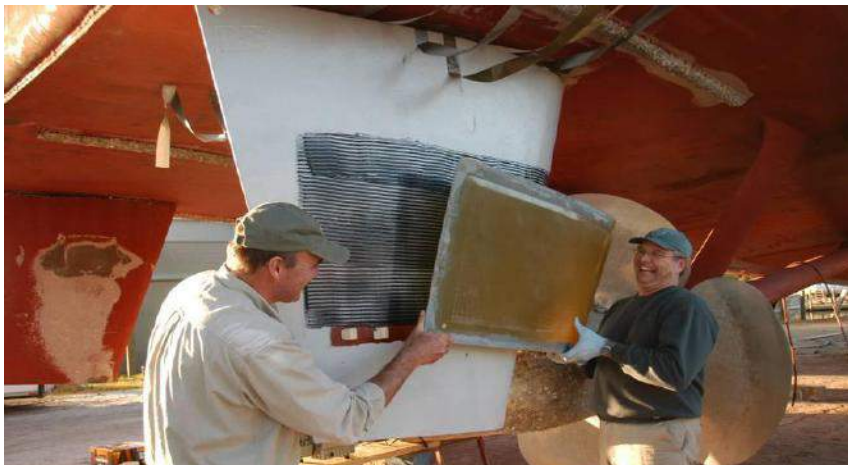
Composite section with Versathane film is placed over notched troweled adhesive on MIL-P-24441 surface
