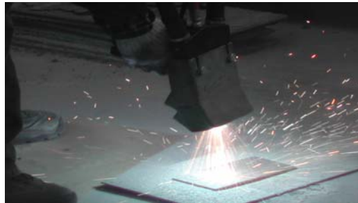
Figure 2.1 - Thermal spray application (From Thermion, Inc.)
